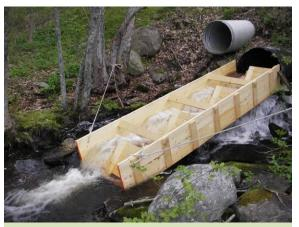
Improperly installed culverts can impede movement and restrict habitat connectivity for many aquatic ecosystems. In this case, a fish ladder may allow some species to traverse the barrier. © Department of Marine Resources
